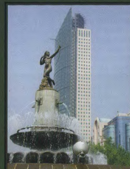
Torre Mayor – Latin America's tallest building developed by the Toronto company Reichmann International.
