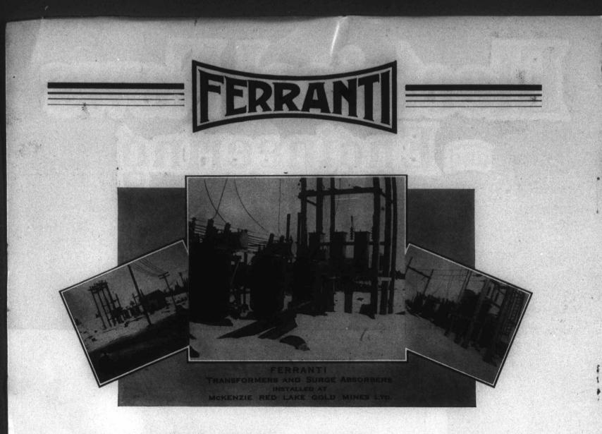
When lightning comes, your electric power must not fail. Ferranti Surge Absorbers give complete protection to properly designed transformer windings. They are particularly valuable in mining districts where solid rock makes ground resistances high. The resistance of the ground is not an important factor in the effectiveness of the protection by the Surge Absorber.
