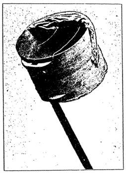
The above is an illustration of the Alpaugh Swarm ('atcher. To the hand'e is attached a cord which may be extended any length and, after the swarm has been shaken into the box, draws the cover over the catcher. The appliance is also away ahead of the Manum Swarming Device as it can be used to jar the tree. Any practical bee keeper will see the immense value of this feature.
