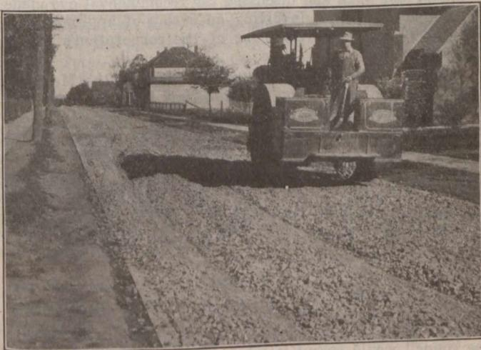
BROKEN STONE BASE FOR BITUMINOUS ROAD, PENETRATION TYPE, MIMICO, ONT., SHOWING DEPRESSED CURB
