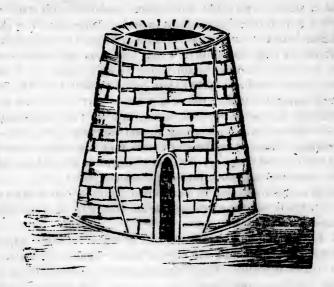
The bore or hollow of the inside should diminish in size from the top of the archway downwards equal to one half the diameter at the bottom. The kiln must be built of rocks that are capable of enduring a strong heat. Clay slate, grauwacke,
