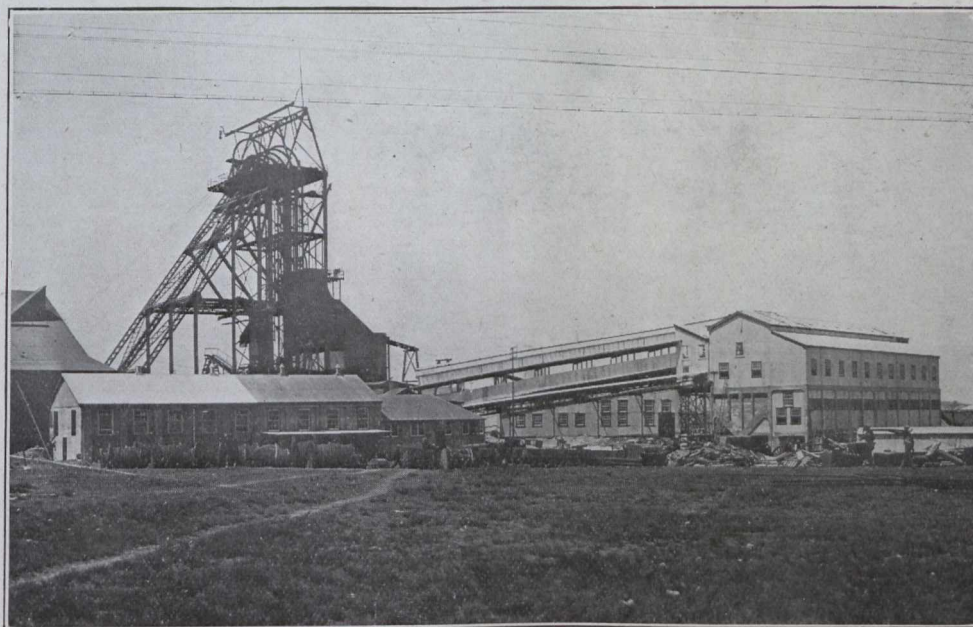
No. 2 Shaft, Sorting and Crushing Station.
