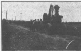
Consolidating the Metal
