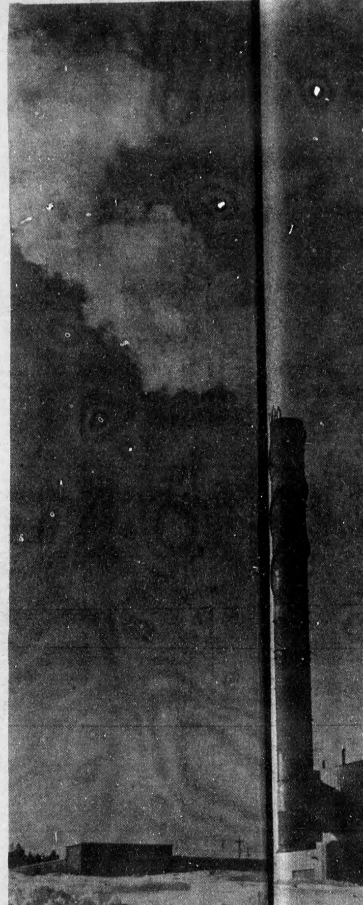
THE NEW UNIVERSITY HEATING PLANT IN MONTGOMERY
