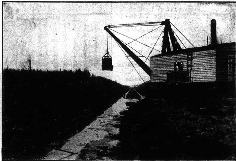
Drag Line Shovel at Work, Edson, Alta., G.T.P. Railway.
