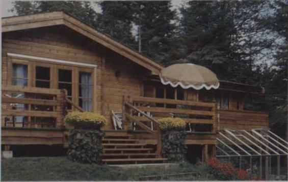
Pan-Abode Buildings of British Columbia sells pre-cut, 3" by 6" and 4" by 6" logs which you can stack up into a handsome, quiet and long-lasting house.
