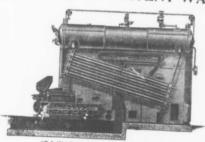
B & W. PATENT WATER TUBE BOILER
