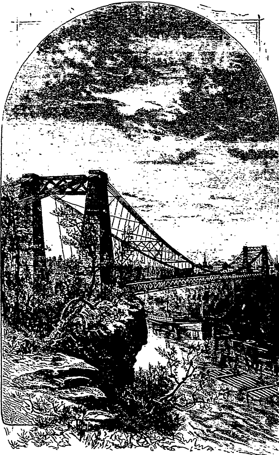
SUSPENSION BRIDGE, FALLS OF ST. JOHN RIVER, ST. JOHN, N. B. Specimen of 250 cuts in "Methodist Magazine" for 1884.
