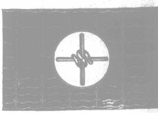
Large (No. 9) hard steel wire is used throughout. The lock makes a joint that cannot be moved.
