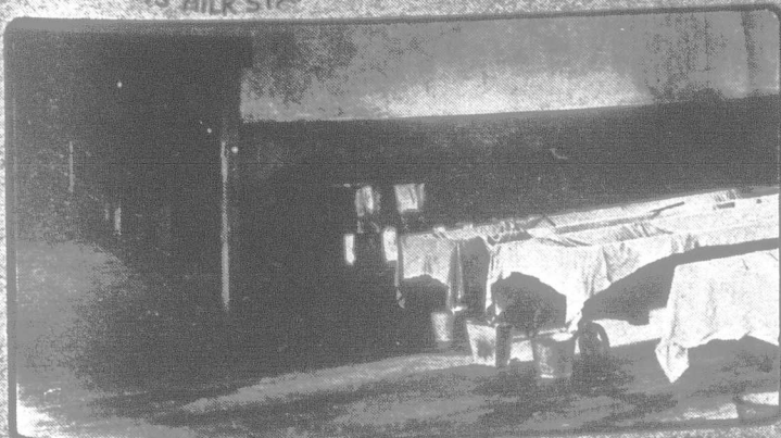
THE MAKE ROOM OF A PERTH COUNTY FACTORY
