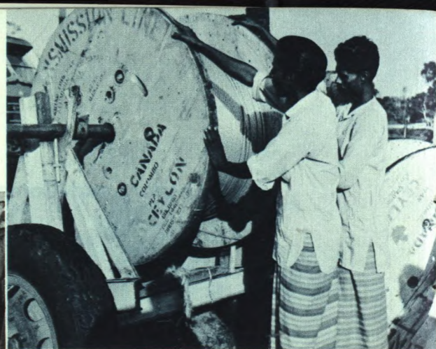
Unwinding cable at the Gal Oya Project in Ceylon.
