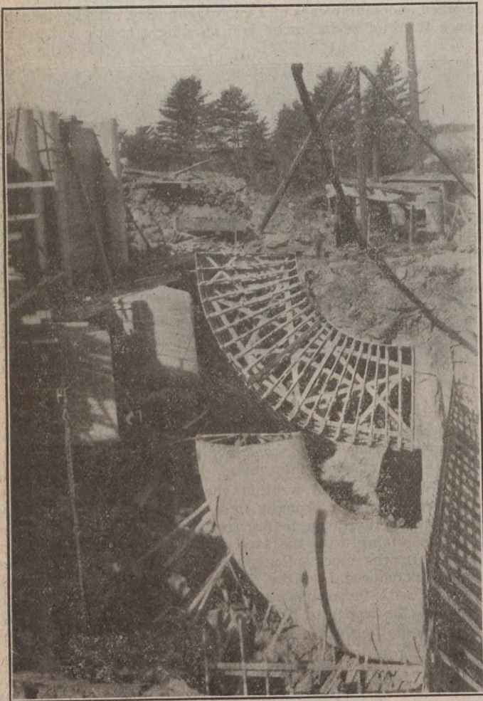
PLACING FORMS FOR DRAFT TUBES
