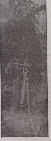
The CC-21 illustrated here, is the result of many years experiment in stoping drills. The control is simple—only one control handle—the drill is not heavy on the runner, pressure on the air feed can be varied for the starting of holes; the machine is powerful, but does not burn the steels; the air consumption is low, and the u p k e e p bill unusually small. 1
