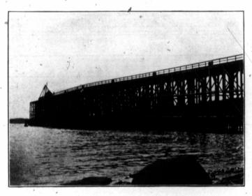
Coal Shipping Pier in Sydney Harbor, in course of construction. Coal from this pier will be delivered direct from railway cars through chutes to ship's hold.
