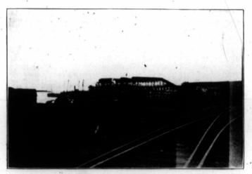
Coal Shipping Pier in Louisburg Harbor, showing overhead travelling way of belt conveyor, used for carrying coal from storage pocket to point of shipment.
