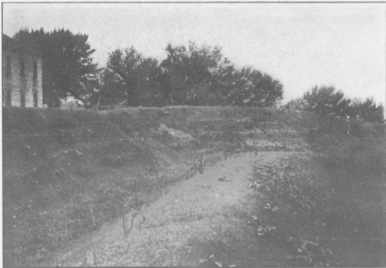
THE NORTHWEST BASTION.
