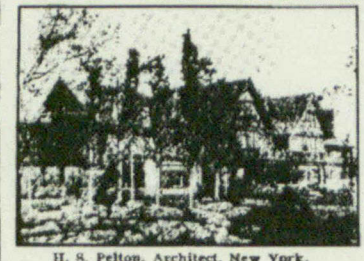
H. R. Pelton, Architect, New York.
