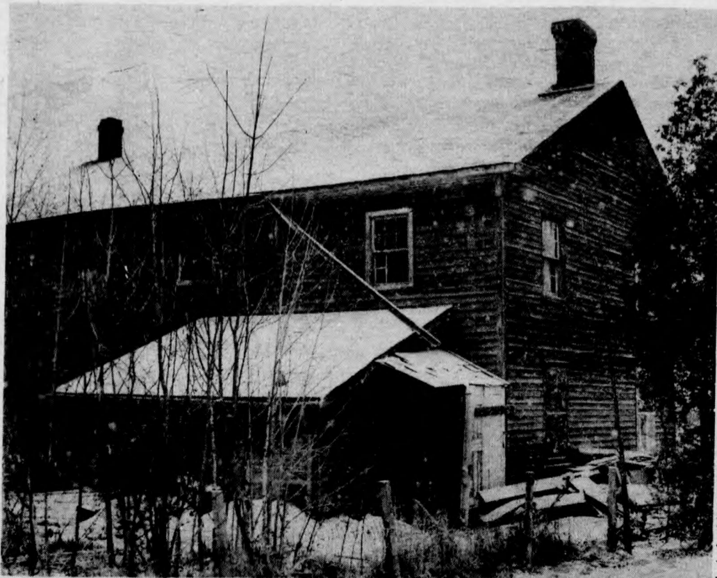
Green Bush Inn just prior to demolition.
