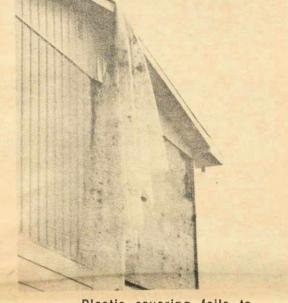
Plastic covering fails to remain on units roof
