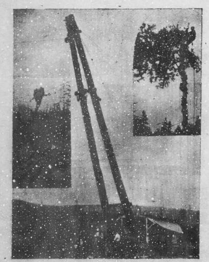
Picture of "A" frame showing, at top, sky-line, and, immediately below, main-line. At centre, on cross-piece, is the haulback: the other lines are the guy-wires. Left: carrage, showing pulleys, position of cables, and chokers attched to logs. Bight topping a birch for a spare-tree.
