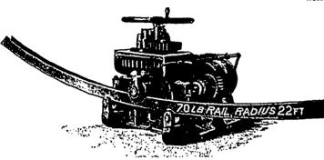
The weight of this machine, as shown in the above cut, is about 3,400 pounds. A lighter kind is made for railroad rails only, and can be mounted on a platform car and connected by a six-inch belt with any seven or eight horse-power engine resting on the same car and fed from the locomotive. The rails can be fed from a car in the rear, through the bending machine, on to another car in front, where they are ready for the track layer. These machines are built also
