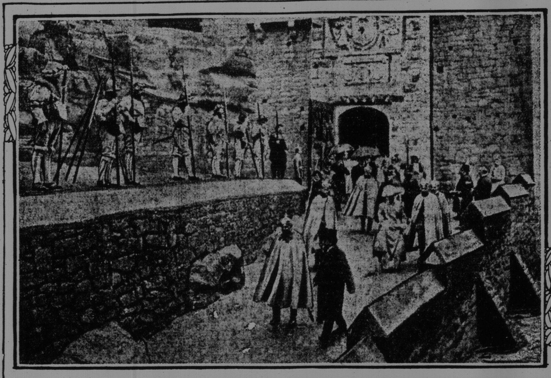
REPAIRS MADE AT THE REINTEGRATION OF THE CHANCEL OF LEPOVA
