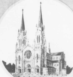
The New Basilica St. Anne de Beaupré (Under Construction)
