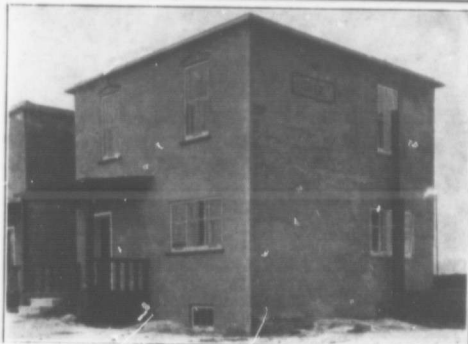
A workman's home, built entirely of concrete. The walls have continuous cavities, a unique feature in this kind of building
