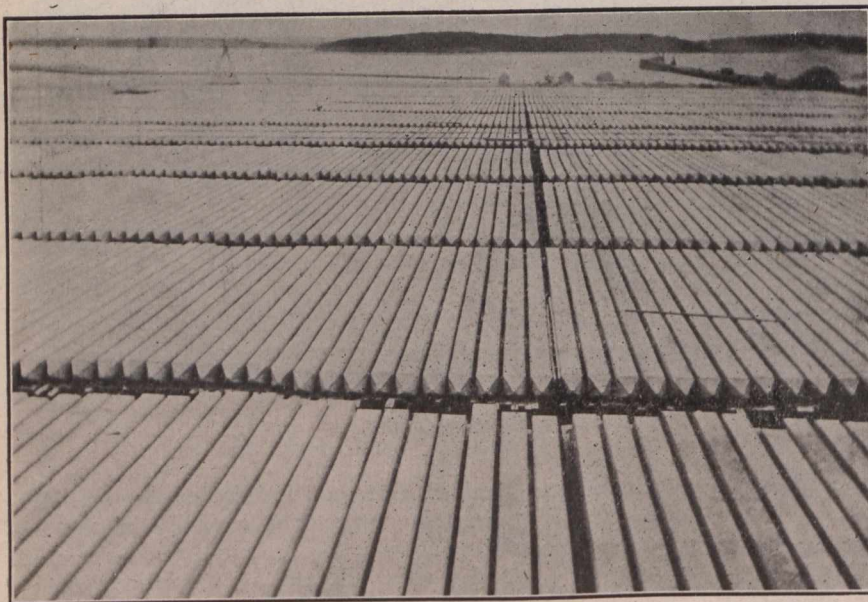
Fig. 4.—View of Pile Casting Yard.
