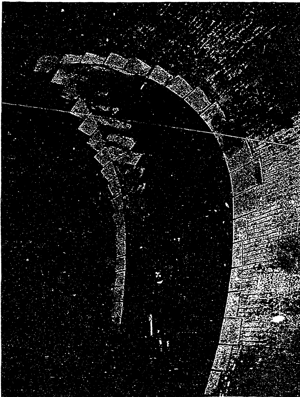
JUNCTION OF HORSESHOE TUNNELS. WATER POWER AT NIAGARA FALLS.
