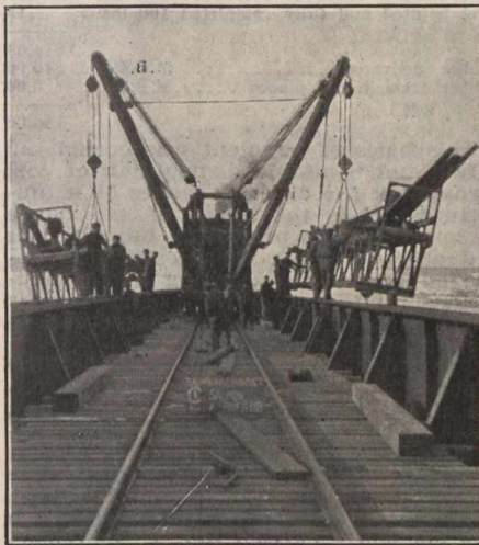
Fig. 7—Method of Raising and Moving Rivetting Galleries.
