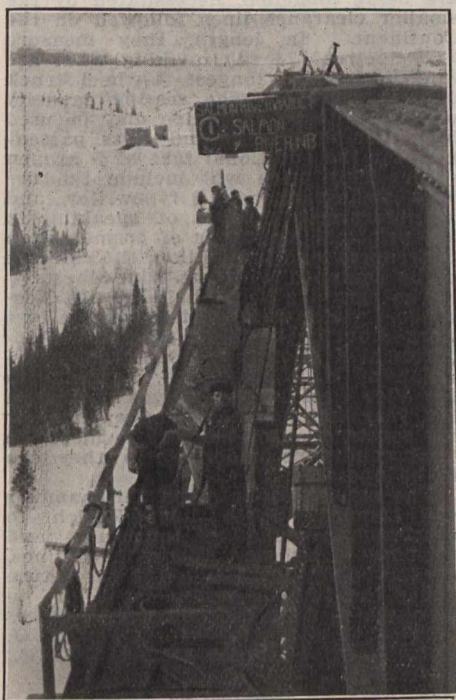
Fig. 8—Rivetting Gallery in Position at Top Tower.
