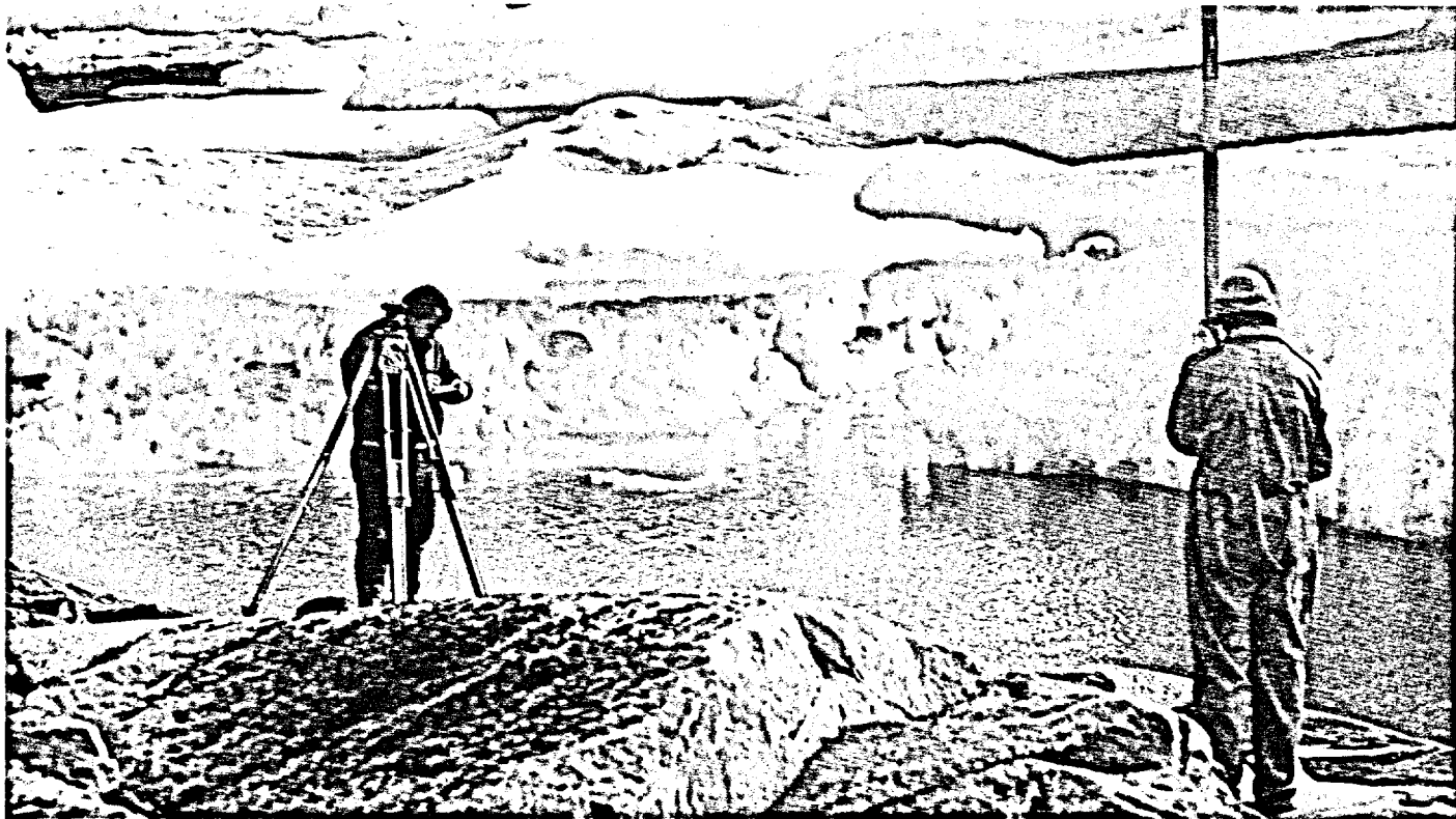
Installation of a marigraph for tidal studies: Fury and Hecla Strait, Northwest Territories.
