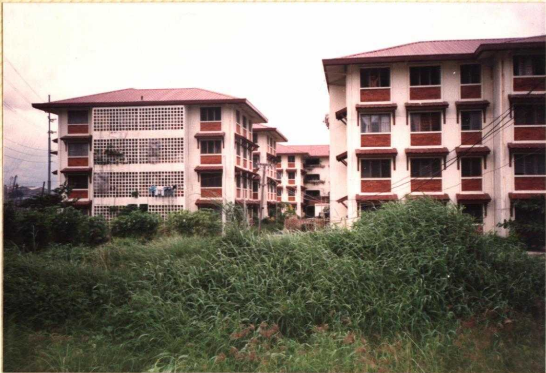
No. 49. A BLISS Guadalupe block partially occupied.
