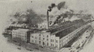
NEW FACTORY BUILT IN 1895 SINCE THEN THE FOLLOWING EXTENSIONS HAVE BEEN MADE MACHINE SHOP LENGTHENED 140 FT NOW 440 x 125 BOILER SHOP 100 FT NOW 220 x 60 1 WITH CORRESPONDING INCREASE MOULDING SHOP 100 FT NOW 180 x 80 1 IN EQUIPMENT BLACKSMITH SHOP 40 FT NOW 100 x 40 1 IN EQUIPMENT
