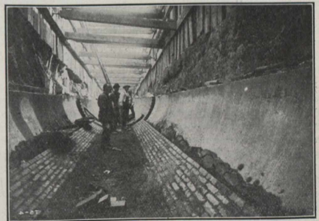
High Level Interceptor, Open Trench Work.
