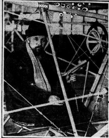
HELICOPER SETS NEW FLIGHT MARK A new record was set by the de Bothezaat helicopter, being perfected The machine, which by the U. S. air service at McCook Field, Dayton, O. rises and descends vertically, reached a height of 15 feet and remained in the air two minutes and forty-five seconds. Professor de Bothezaat
