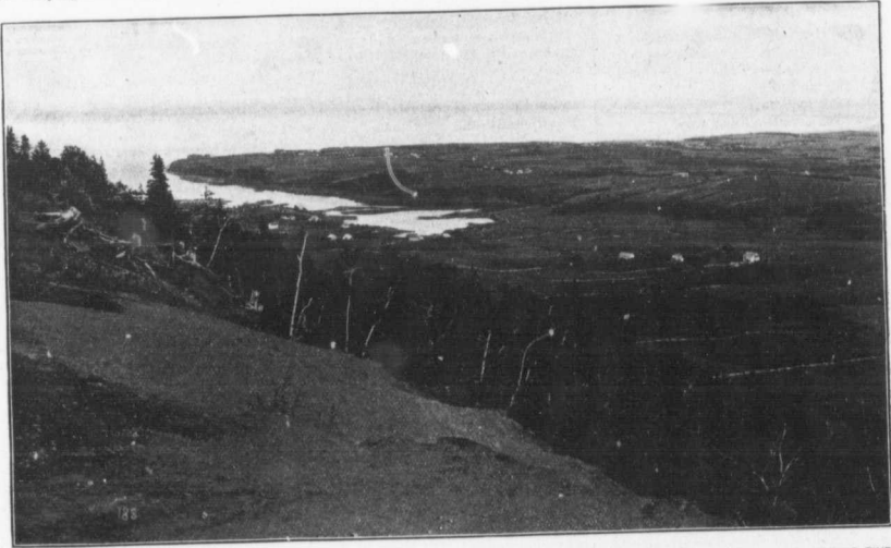
VIEW FROM "LOOK-OFF POINT," OVERLOOKING FIVE
