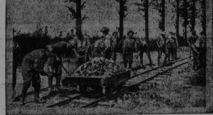
Canadians laying a light railway track near the firing line. The permanent way was made up with ballast provided by demolished buildings in the neighborhood. The Canadian Railway Corps was organized by Gen. J. W. Stewart, railway contractor of Vancouver, and includes in its ranks men from all sections of Canada.
