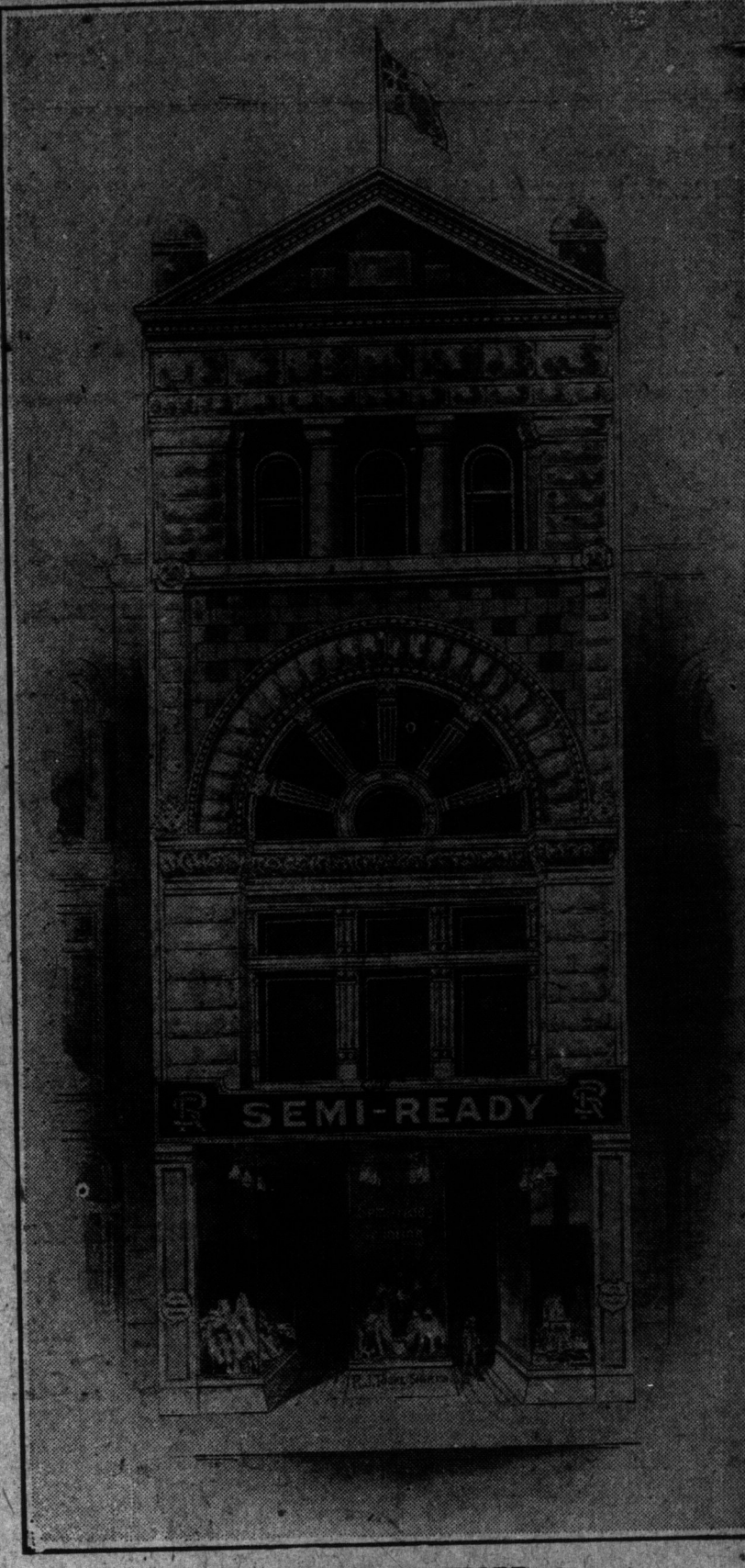
THIS IS THE STORE and the four-storey building at 143 Yonge street, which we will submit to the highest bidder for six and one-half years. Semi-ready, Limited, Montreal, or any reputable real estate agent. Particulars on the premises.
