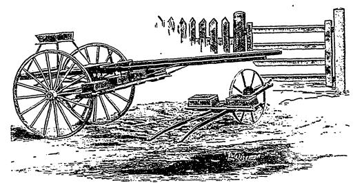
The above cut represents our patent poison Distributor for Spreading Paris Green and Plaster on the potato bug. It is made to use by fland or Horse Power. The Hand Machine is intended to take two drills at a time, and the Horse Machine four s. So that the labor is reduced to a small affair. It has been ten years in use, and has given good satisfaction. It saves your green, and therefore your money.
