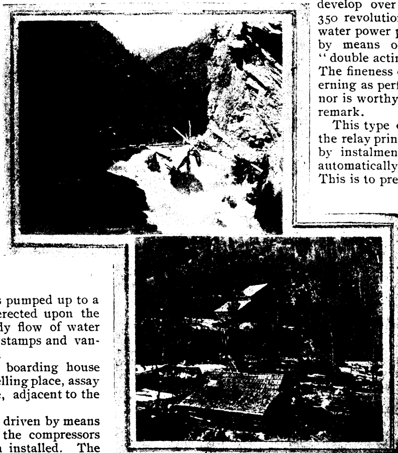
1. THE DAM AND FLUME.
