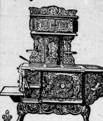
The important feature of this system is the diffusive flue which draws in fresh air, superheats it and distributes it evenly throughout the oven. The article on the bottom shelf farthest from the fire is getting as much heat on all sides as the article on the top shelf next the fire. We would like to explain this more
