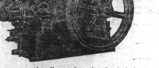
The Jumbo is an exceptionally good engine for hoisting, sawing, etc. Positive starting magneto eliminates batteries and coils and their attendant trouble.
