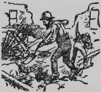
"I WAS HELPING TO DIG OUT THE CELLAR."
