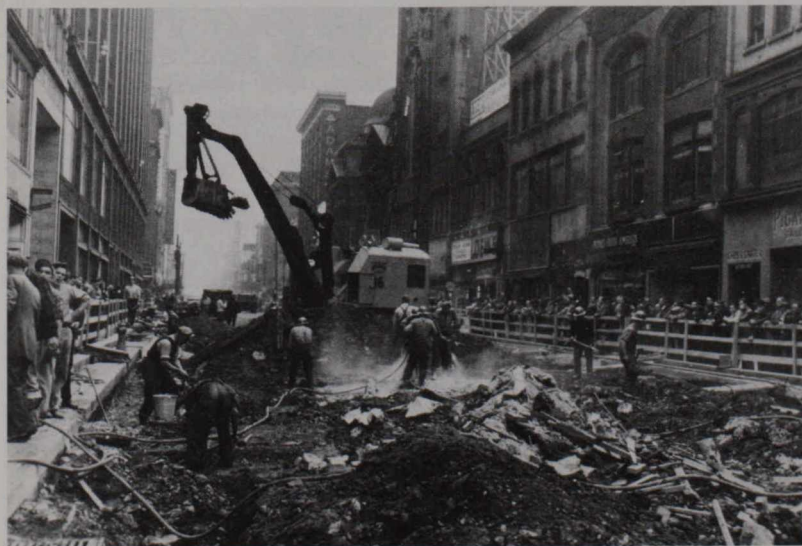
Digging up Yonge Street to build the subway, 1950.
