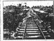
INDIAN RAILROAD AFTER AN EARTHQUAKE fer irritating delays from occasional ground swells, which seem to do no great damage to other property, but are especially disastrous to railroad tracks. This unheralded twisting of rails is one of the drawbacks to rail roading in India.
