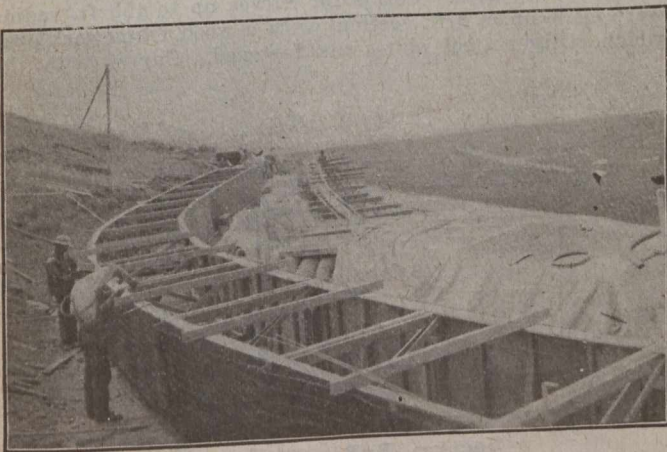
FIG. 1—CONSTRUCTING THE FORMS
