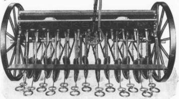
grain box is supported by an I-beam, and this I-beam carries the separate axles, which are short and of ample strength for long wear. The result of this even sowing at even depth in close drills is shown in the growth of crop and its quality, with drought protection impossible in more open sowing.
