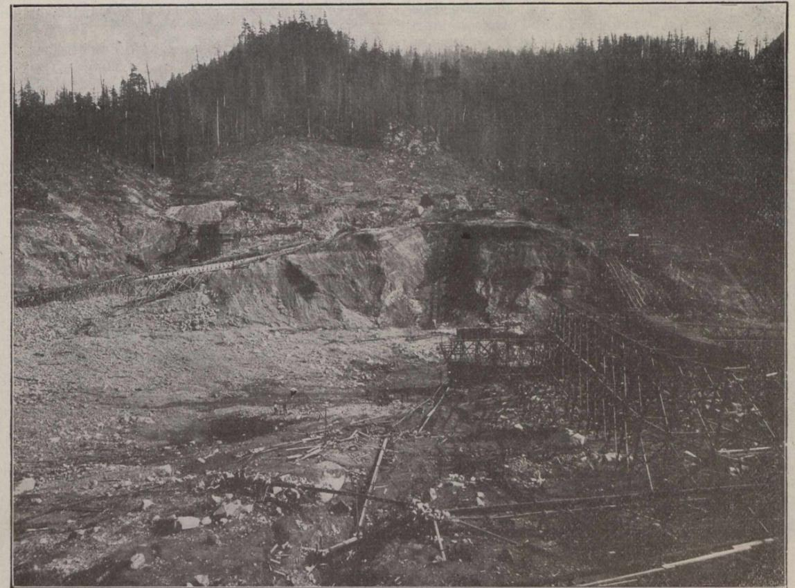
Fig. 4.—Foundation Ready for Hydraulic Filling, Coquitlam Dam.
