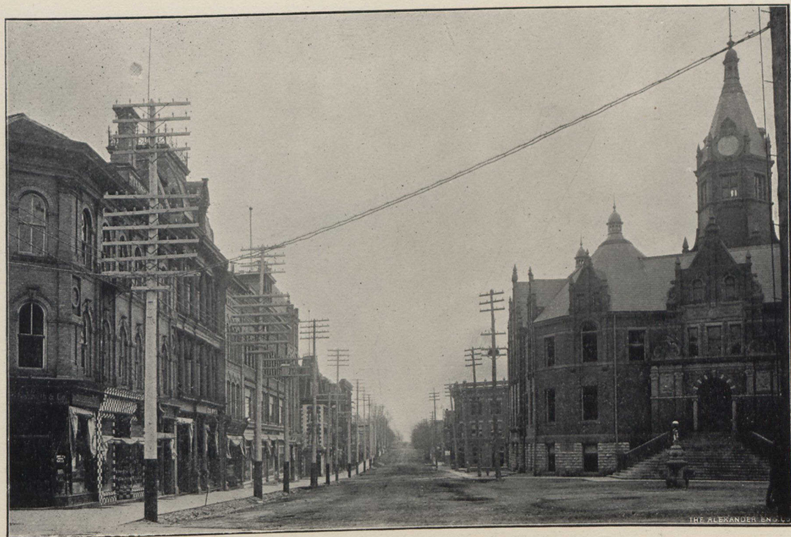
AN EARLY MORNING VIEW ON DOWNIE STREET
