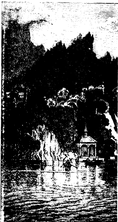
TELL'S CHAPEL, SWITZERLAND (PART OF CUT).
